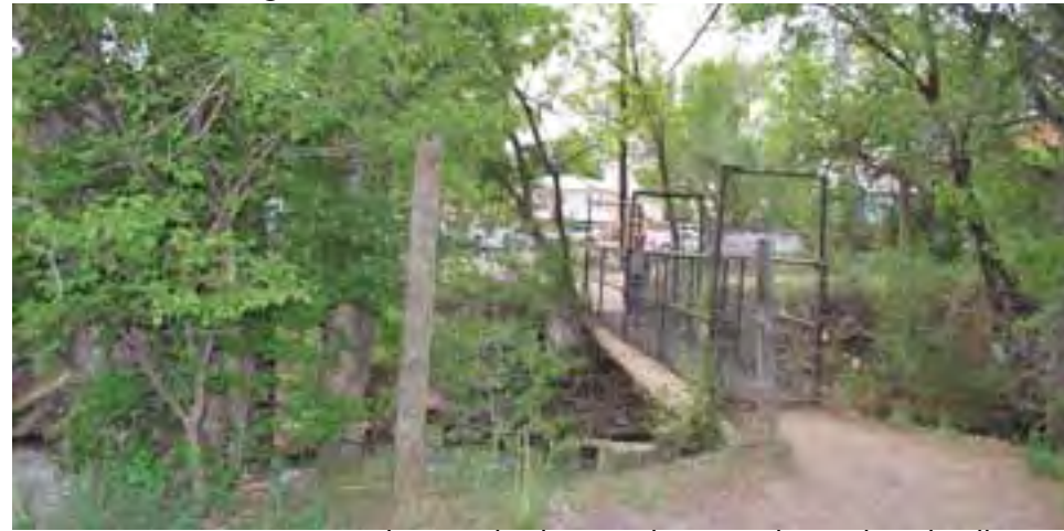
Existing pedestrian bridge at Library, to be replaced Fall 2012
