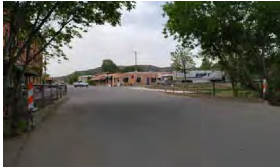
Existing Main Street Bridge
