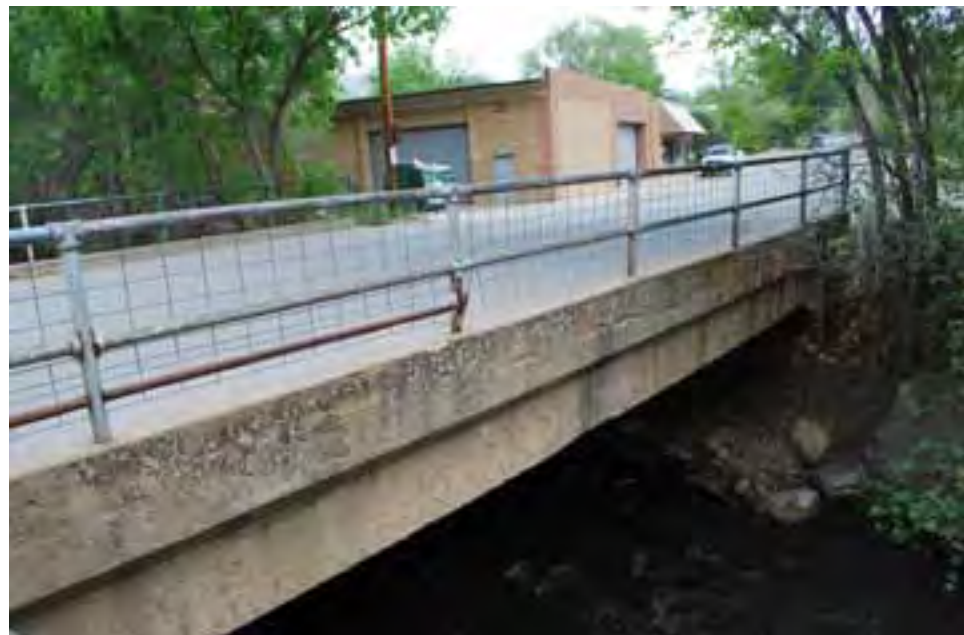
Existing Main Street Bridge
