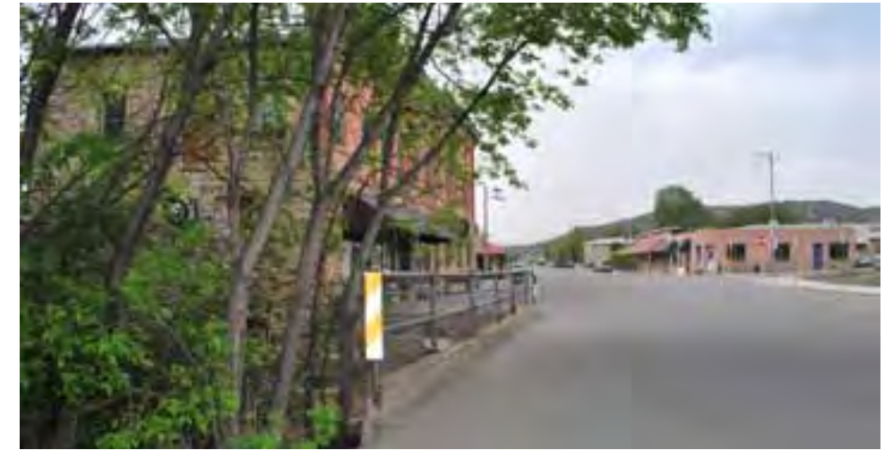
Main St. Bridge
