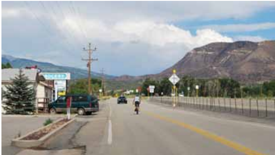
Pedestrian/bicycle facility is needed along the north side of Highway 160. The street is narrow and there is no safe place to ride or walk.
