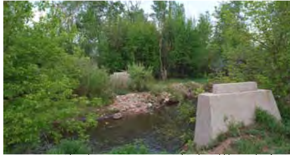
Bridge abutments in Cottonwood Park could be used in future
