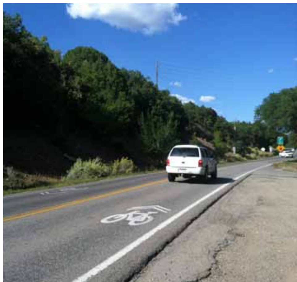
A 'share the road' symbol could be painted even if the road is not wide enough for a complete bike lane.
