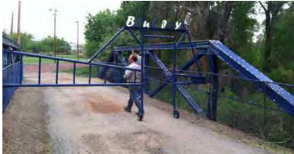
Pedestrian bridge on school property
